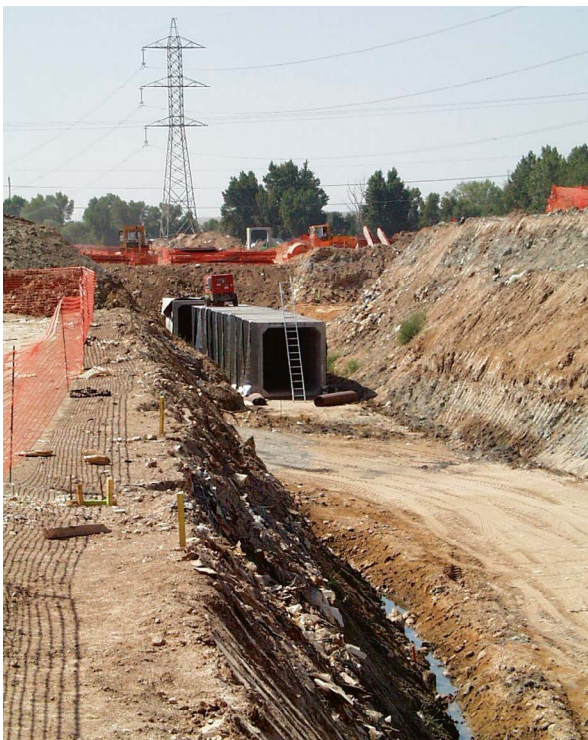
Cut and cover tunnel installation in mainland Europe
