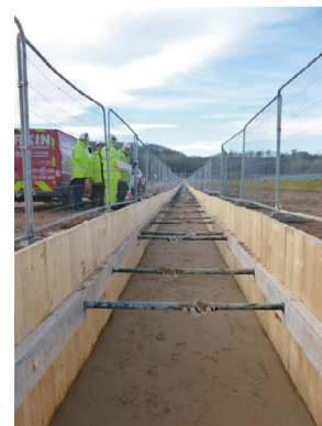
Cable joint bay on a directly buried cable
