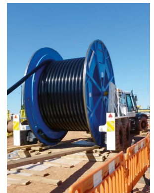
Cable drum offloading cable on site
