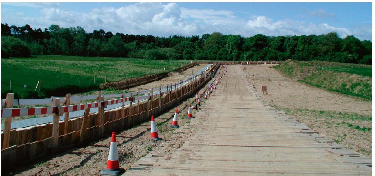
A cable swathe during construction with a single cable trench open
